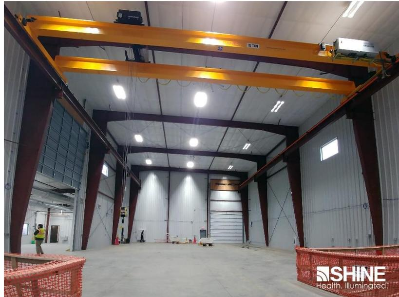
*Photo: 15-ton crane inside Building One.*
